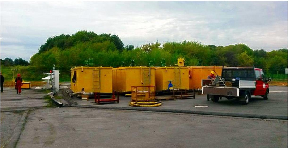
*Figure 45. Installation of the storage tanks with 35 m<sup>3</sup> capacity each. The left tank acts as backup.*
